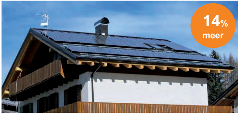
Noord IT / 8,75 kWp
