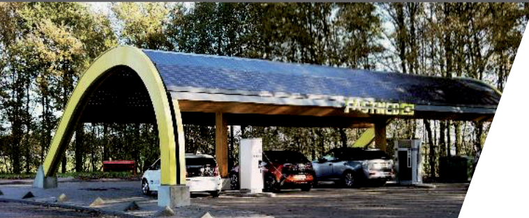
Fastned electric car fast charging stations | 3MW
