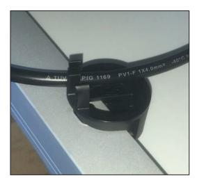
5. Then install the solar panel on the horizontal mounting rails, making sure the installation support hooks behind the edge of the upper mounting rail.
