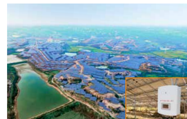
Zhejiang Longyou Agricultural-photovoltaic hybrid PV plant 25MW
