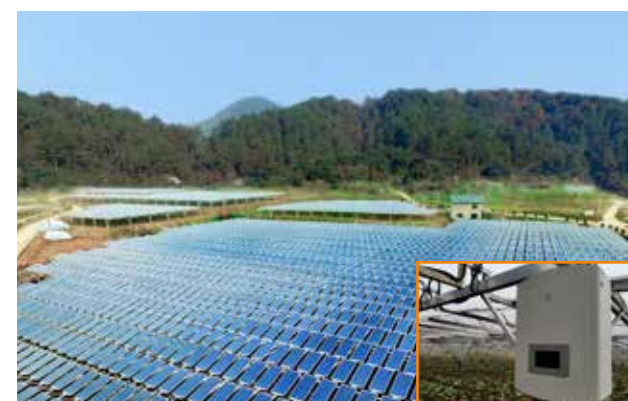
Zhejiang Dajie Agricultural-photovoltaic hybrid PV plant 3MW
