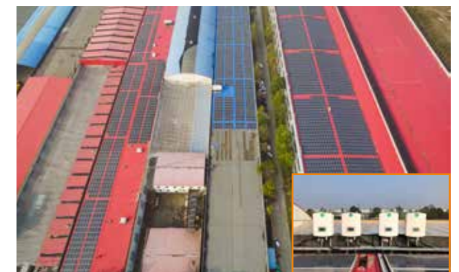
Shandong Weifang Linqupoverity alleviation PV Plant 20MW
