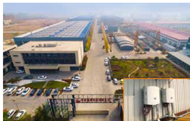
Hebei ZQ Steel 1.5MW
