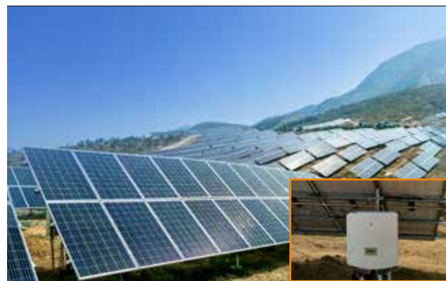
Liaoning Yingkou Jiuzhai PV plant 20MW
