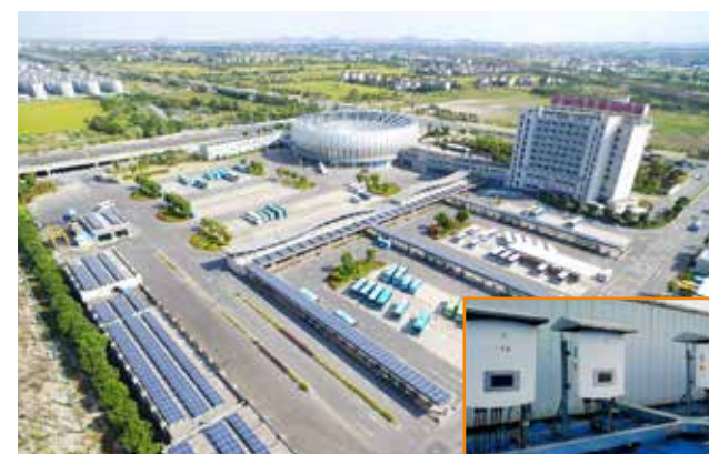
Zhejiang PINGHU Bus Station 472kW
