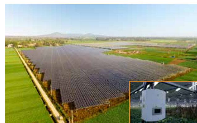
Hubei Guanyin Agricultural-photovoltaic hybrid PV plant 20MW
