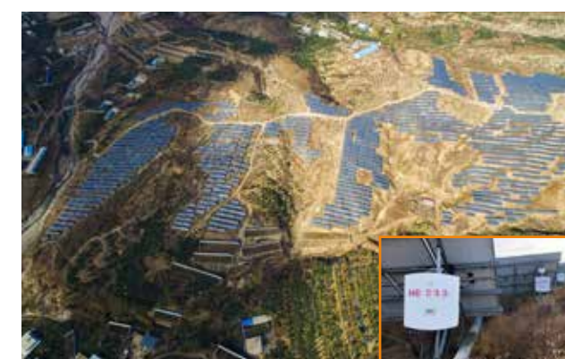
Liaoning Jiuzhai Gaizhou PV plant 20MW
