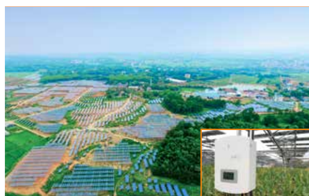
Quzhou Qinghu Agricultural-photovoltaic hybrid PV plant 20MW
