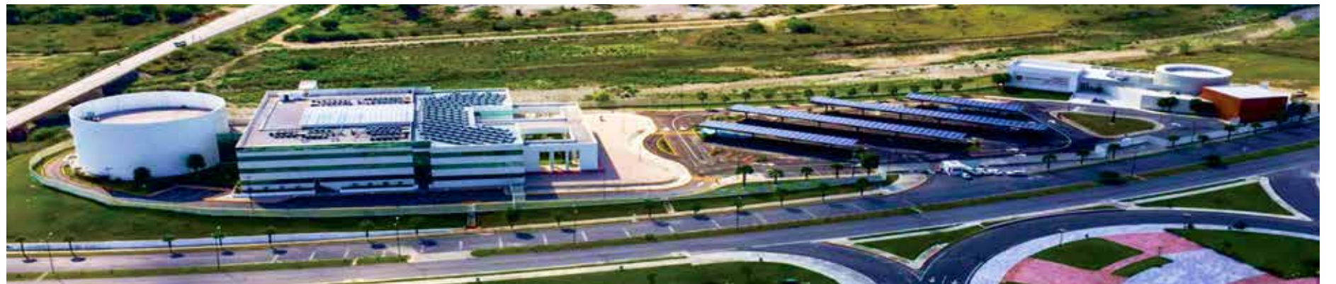
Mexico-Tamaulipas Carport 5MW
